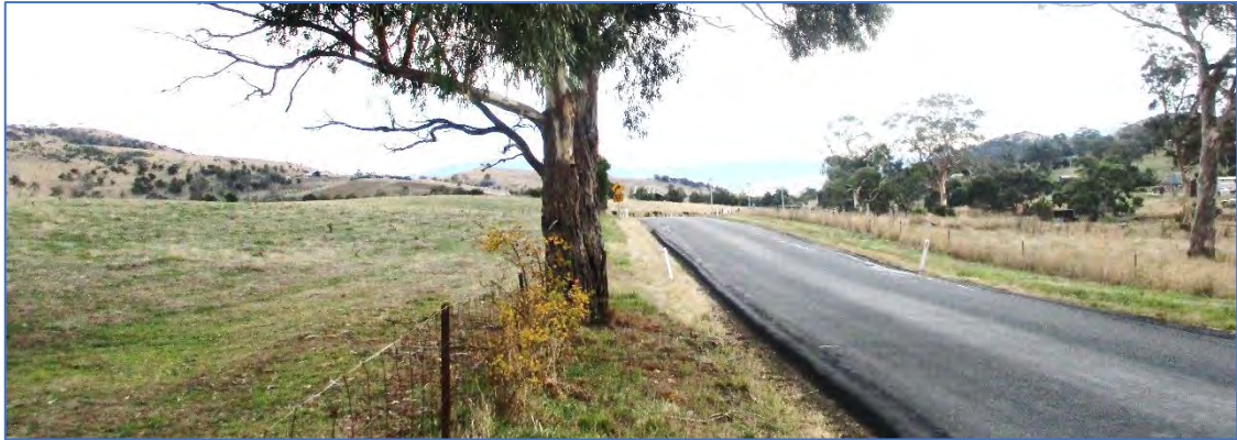
Photograph 6.1B – Available sight distance to the left (exceeding 200 metres)
