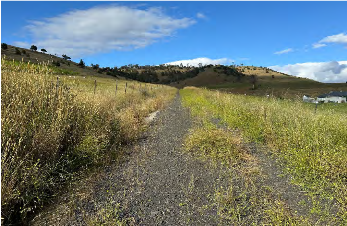
Photo 3: Field photo taken showing existing property access at the entrance with Rosewood Lane.
