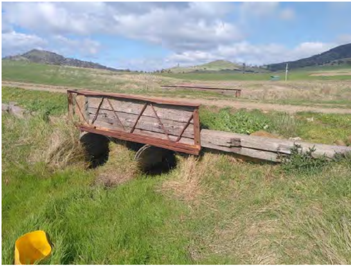
Existing culverts ch 425m
