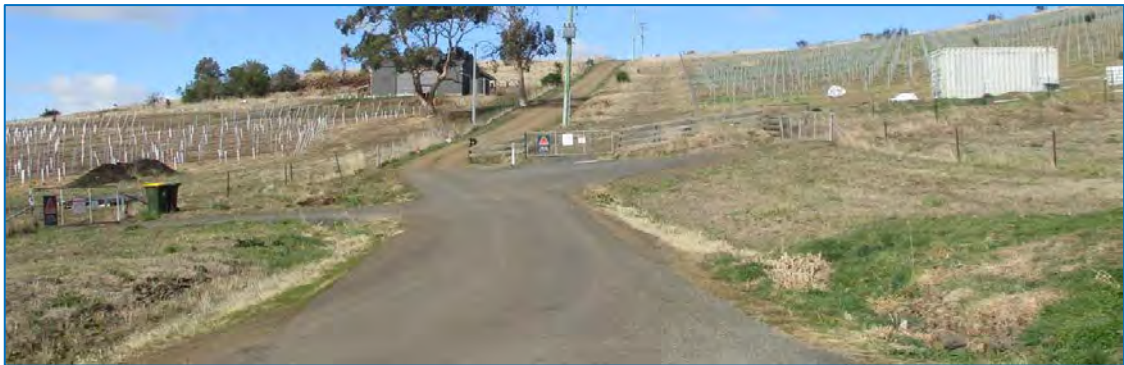
Photograph 6.2 – Available sight distance at end of Rosewood Lane
