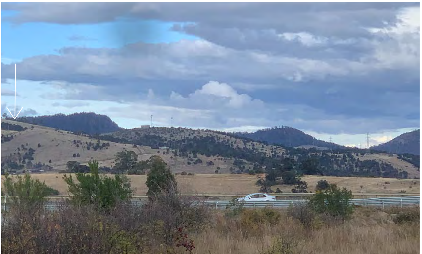
Photograph 8. View from Brighton Transport Hub to the general area of lots 6, 9 and 10. Note the presence of high voltage power lines and telecommunications towers in the broader landscape (Source: Inspiring Place)
