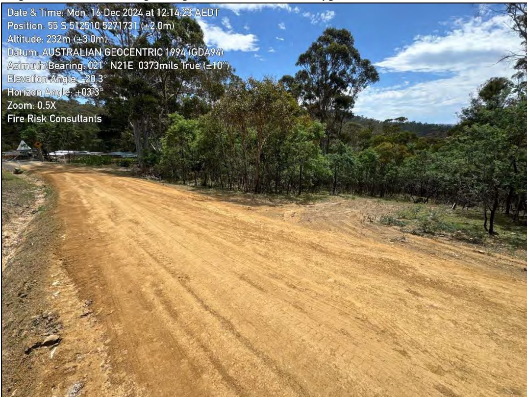
Image 1: Clarks Road - existing turning area recommended to be upgraded.
