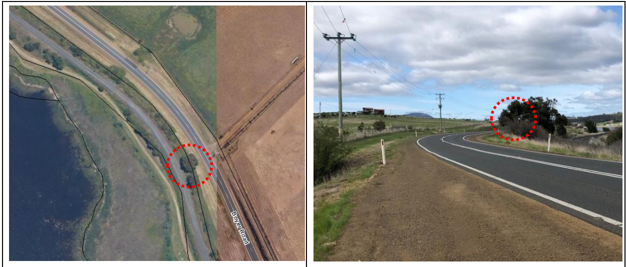
Figure 9 Access 3 Sight Distance - Vegetation Maintenance
