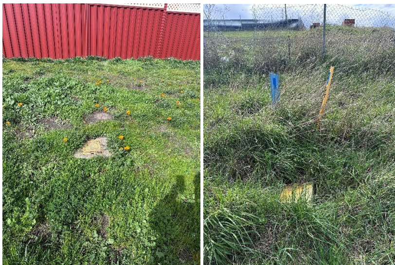
Figure 6 – Existing hydrant (Taylor Cres) Figure 6.1 – Existing hydrant (Cove Hill Road)
