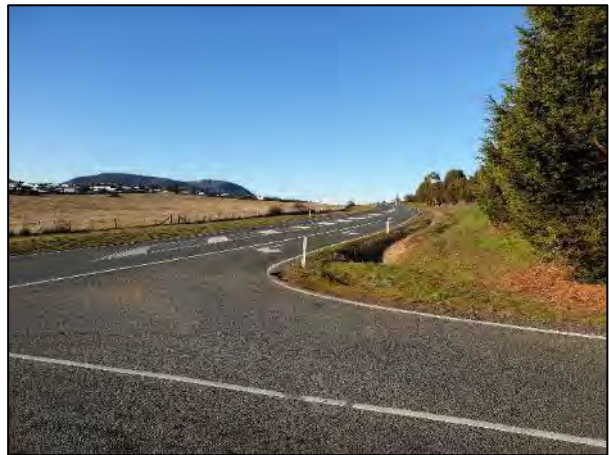
Figure 4 East Derwent Highway looking south
