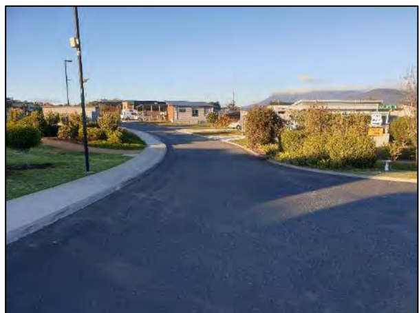
Figure 10 Radius Drive looking south
