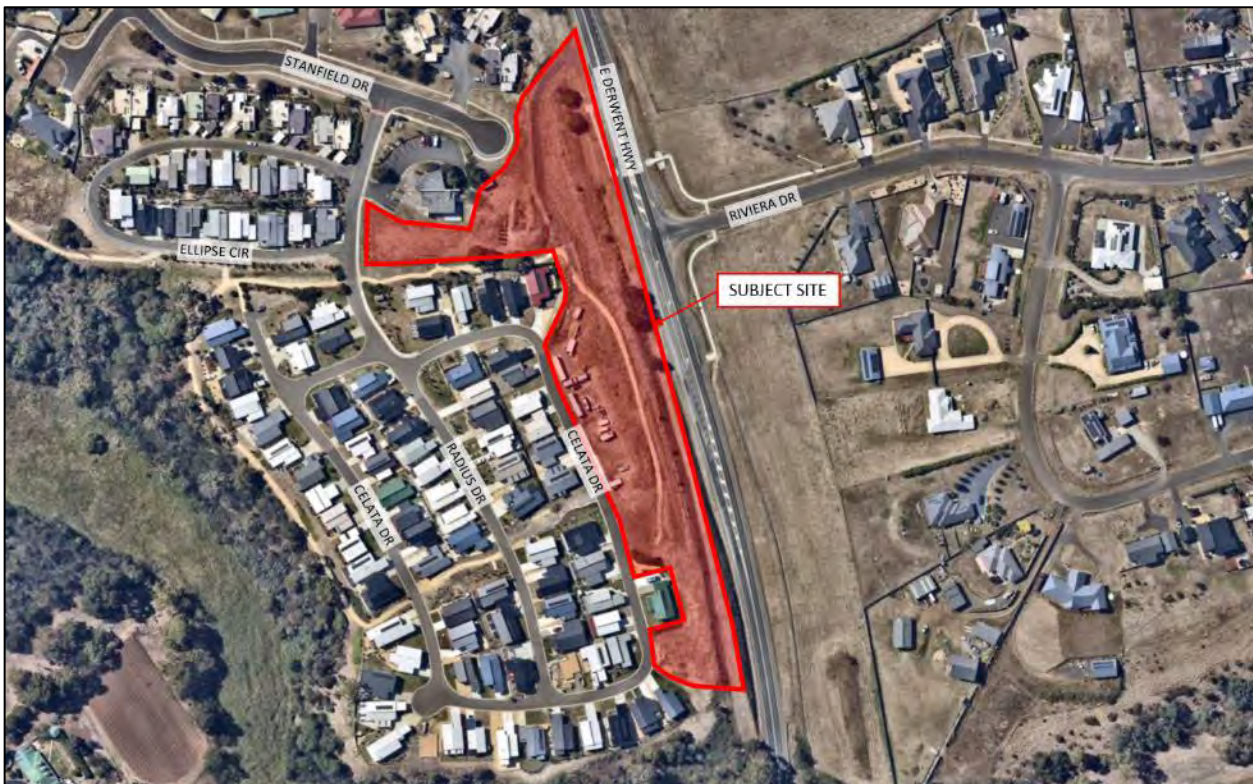
Figure 2 Aerial view of subject site (Source: Nearthmap)
