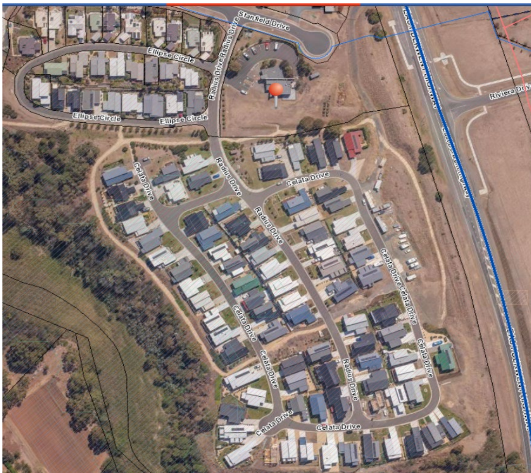
Figure 1: Site plan showing existing development. The proposed development will be sited along the eastern boundary, as shown in Figure 2.
