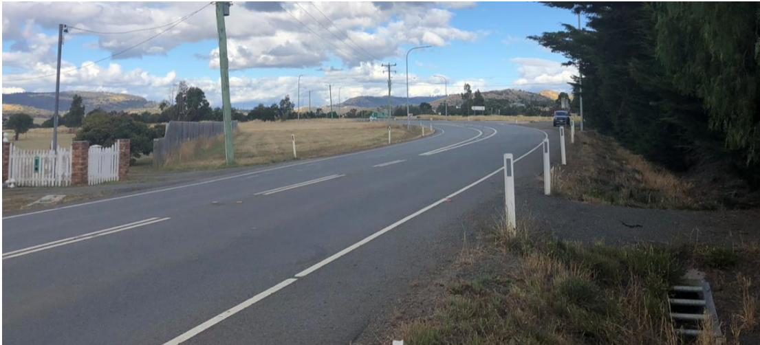
Photograph 5.7B – View looking to the east
