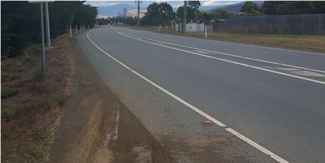
Photograph 6.4A – View looking west from proposed lot 2
