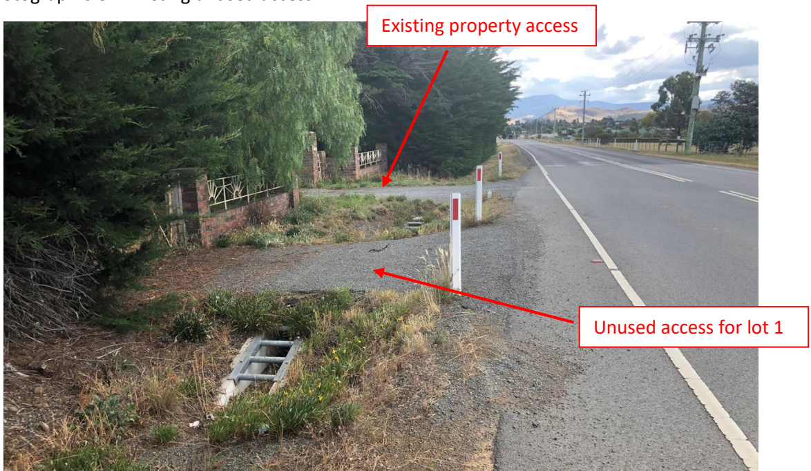
Photograph 6.3 – Existing unused access
