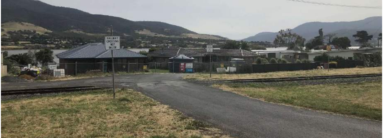
Figure 6 Wallace Street Derwent Valley Line Crossing
