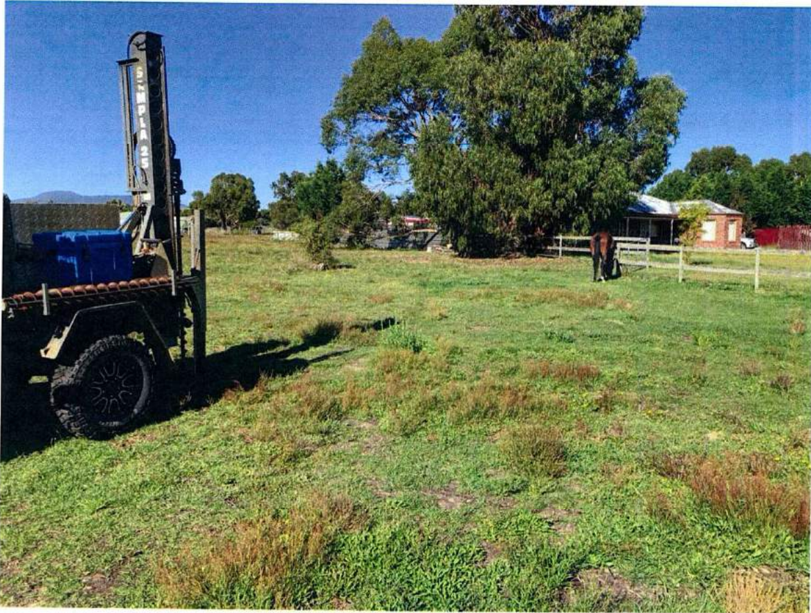
Plate 4 – Lot 2 – Test Hole #1.
