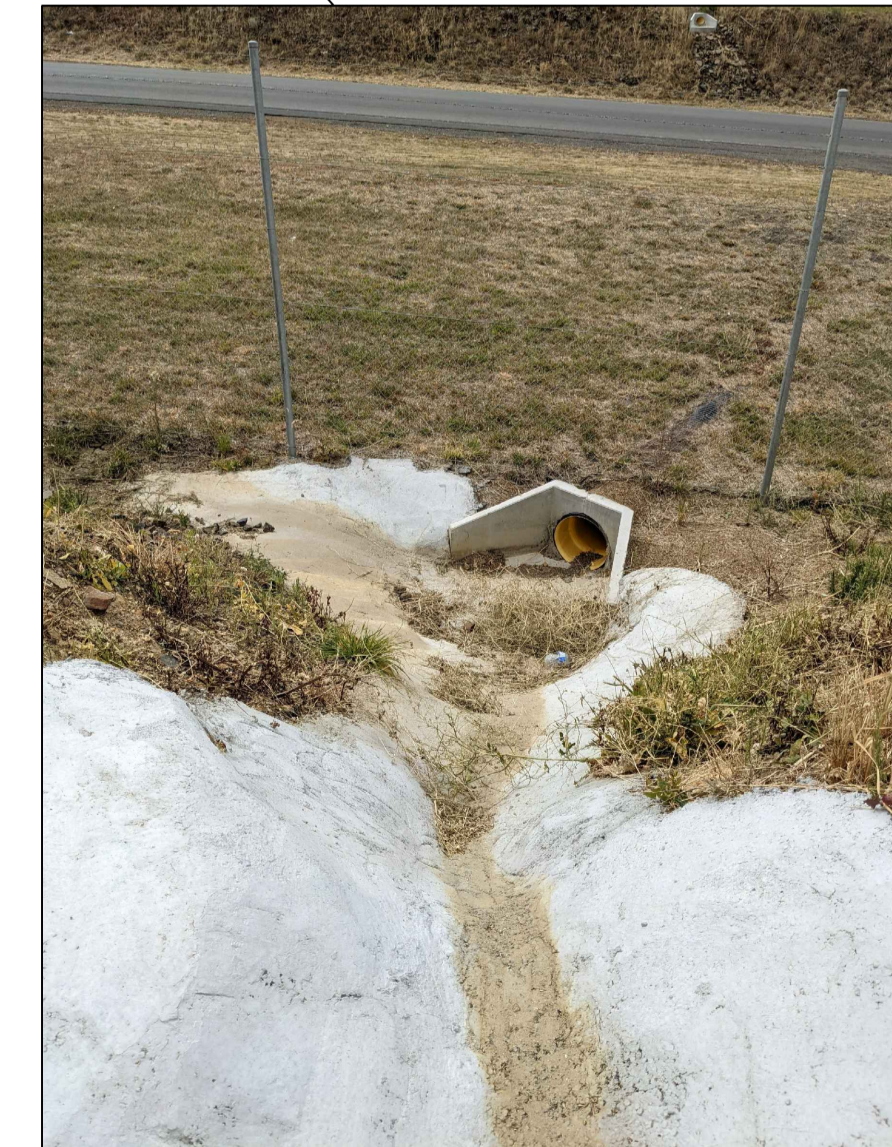
FIGURE 1 EXISTING CONCRETE SPILLWAY & INLET HEADWALL
