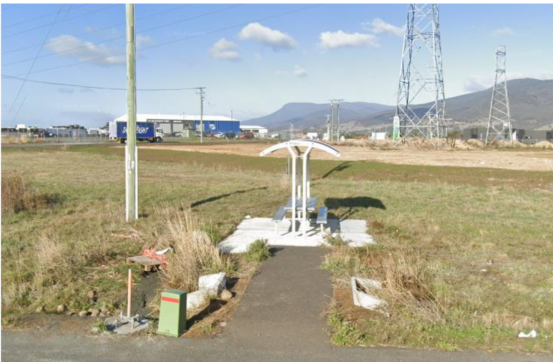
Figure 2 Existing Rest Area
