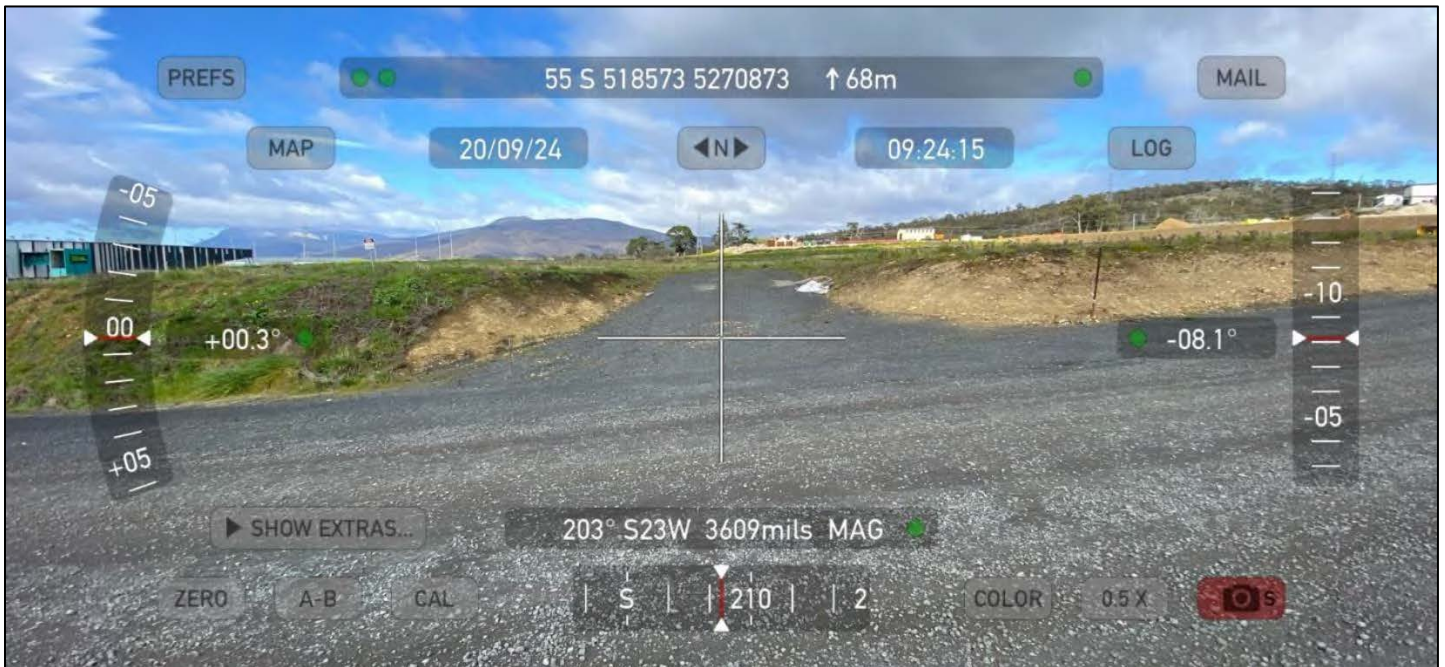
Photo 8: Formed crossover from the proposed new road to the eastern end of proposed Lot 4
