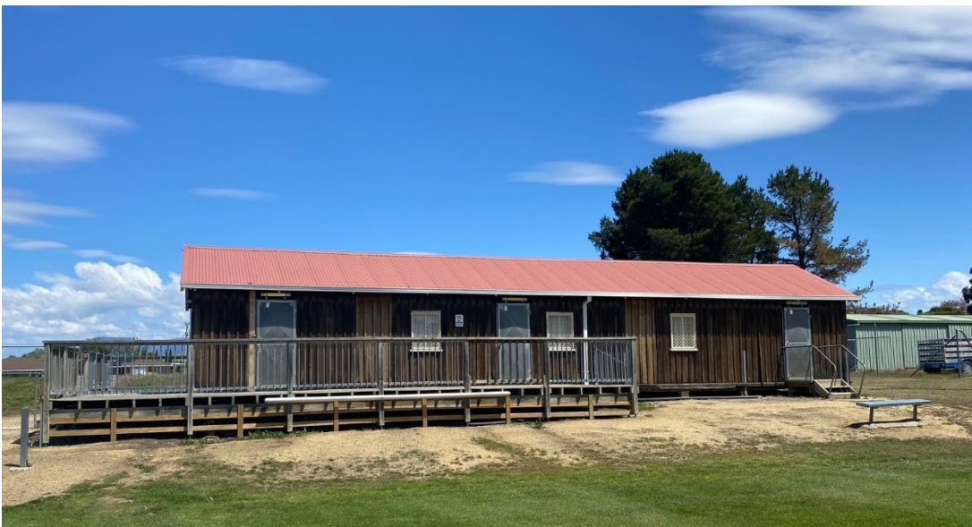
Figure 1: Existing building at Ted Jeffries Memorial Park (Source: Brighton Council)
