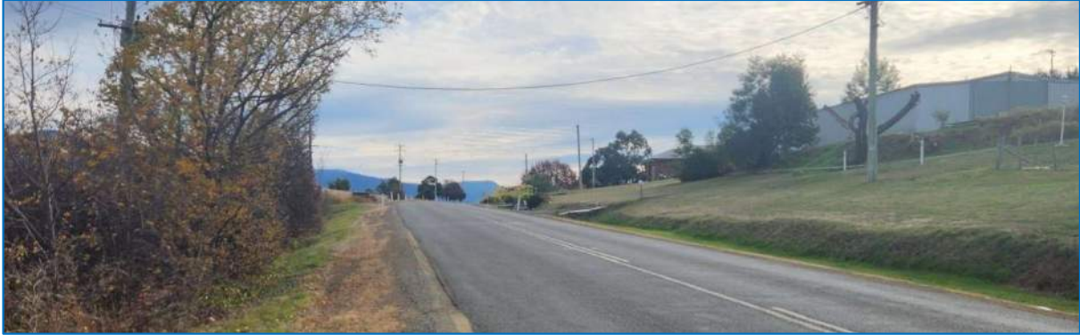
Photograph 12.2 - Available sight distance to the right for lot 103
