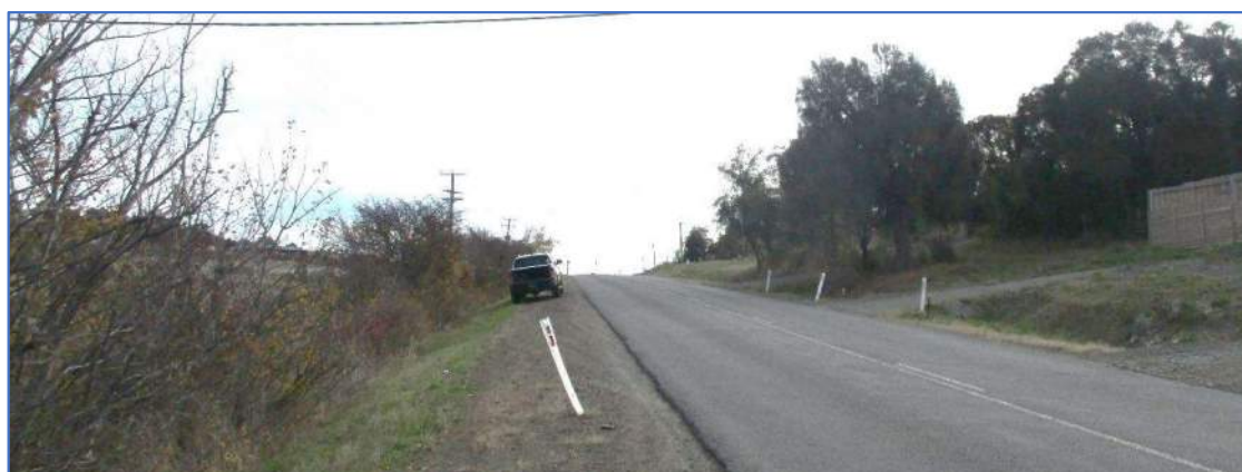
Photograph 8.1A – Available sight distance at the eastern junction to the left
