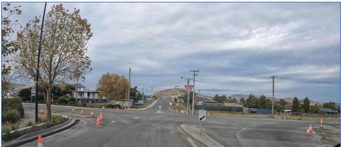
Photograph 5.2 – Brighton Road and Elderslie Road intersection
