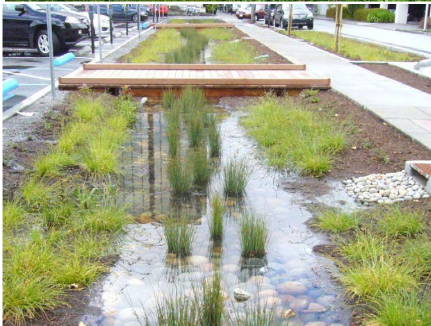
Figure 5 Two different concepts of storm water management utilising rain gardens.
