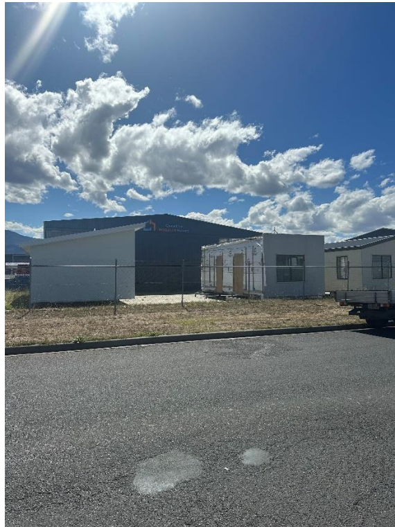
Figure 13 – Existing building and managed land (typical site in this area) west of the property, view facing W, SW
