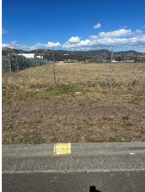
Figure 6 – Existing hydrant (Cowle Road)
