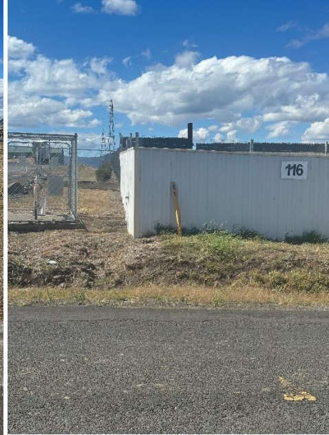
Figure 7 – Existing hydrant (Cove Hill Road)
