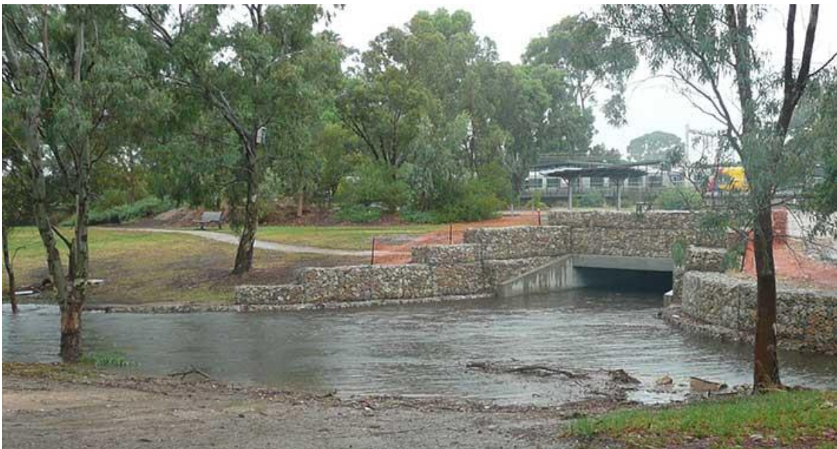
FIGURE 28: UNDERGROUND CULVERT IN BROWNHILL CREEK, SOUTH AUSTRALIA
